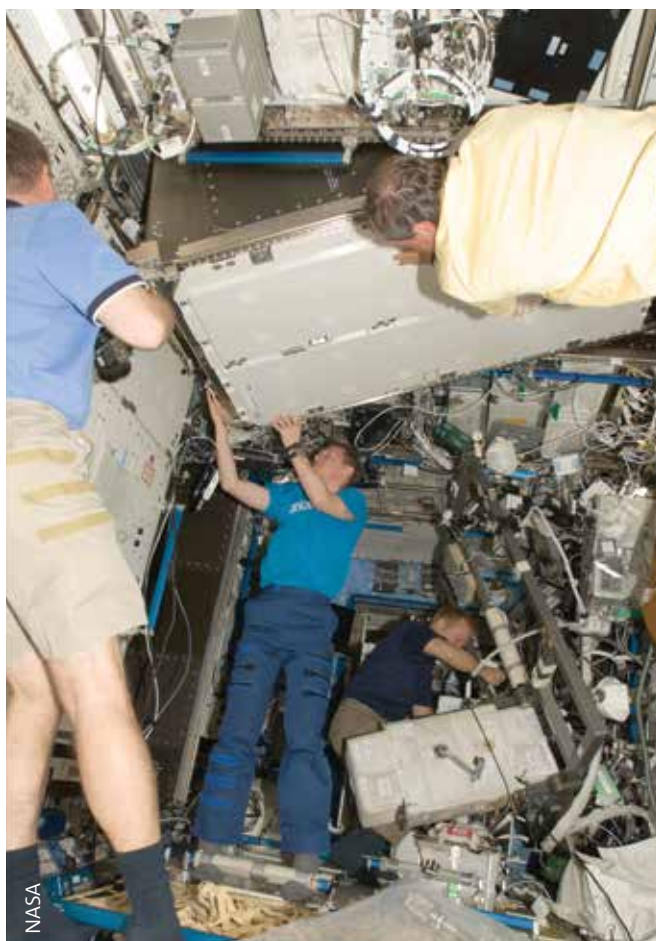
↑ ESA astronaut Frank De Winne (left) and Christer Fuglesang (top right) installing the Materials Science Research Rack which includes ESA's Materials Science Laboratory as its principal payload
